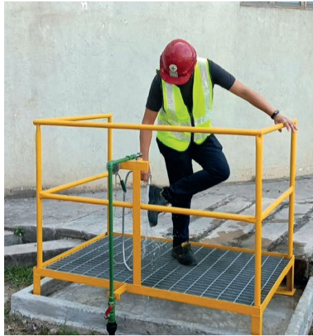
Safety boots cleaning station
