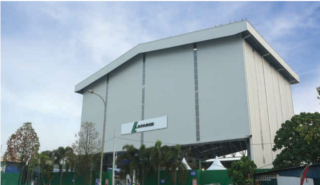
The Chan Sow Lin plant is Malaysia's first enclosed ready-mix concrete batching facility that is built to reduce noise and dust emissions and is capable of reclaiming returned concrete.
